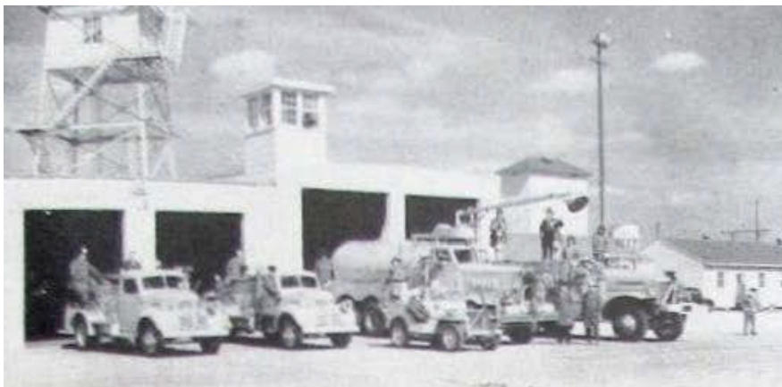
35 Air Engineering Squadron fire department.
